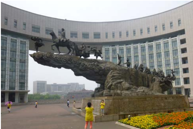
The main building of the National Animation Park in the Tianjin Ecocity.
