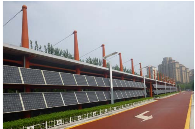
Solar photovoltaic panels along the parking garage of the main administration building at the Tianjin Eco-city.
