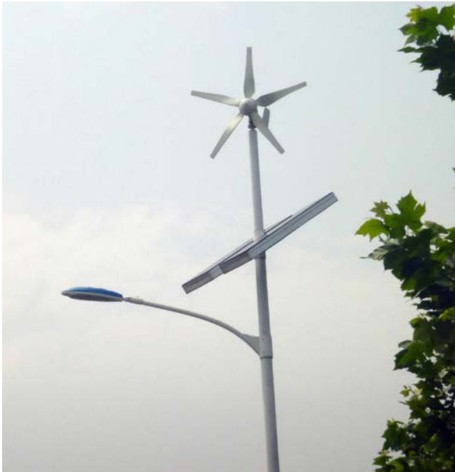
Streetlamps in the Tianjin Eco-city are wind and solar powered.
