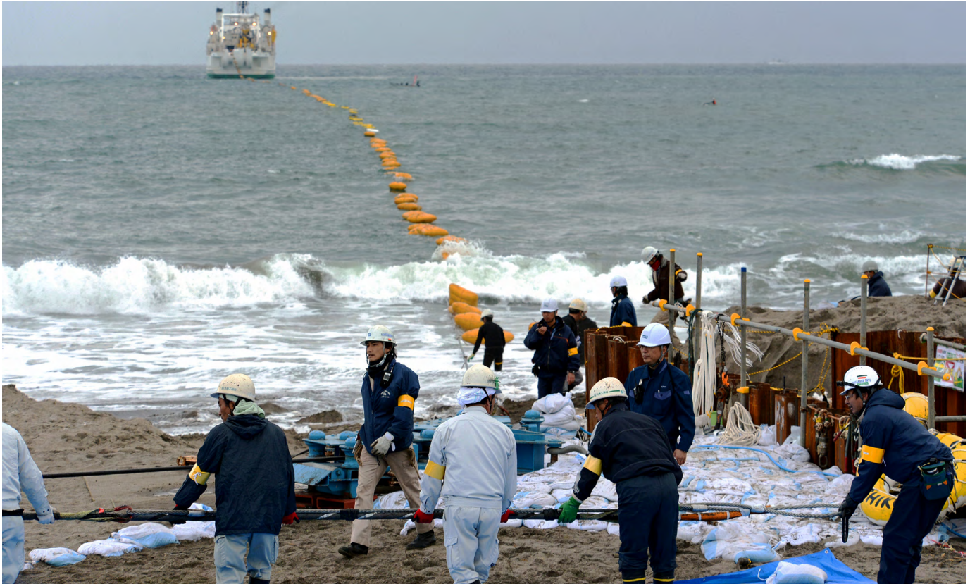
Workers pull an undersea fiber-optic cable from a ship, as KDDI Corp. began an operation to lay a cable connecting Japan and Singapore. Photo by The Asahi Shimbun via Getty Images
